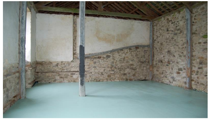
Finished the first coat
